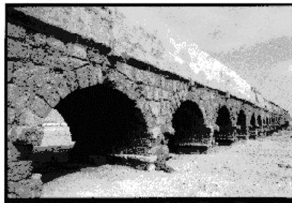
A Roman aqueduct
